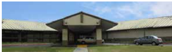
Cornerstone Hospital of Houston – Clear Lake, 709 Medical Center Boulevard
