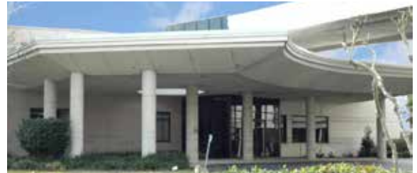
Bay Area Surgicare Center, 502 Medical Center Boulevard
